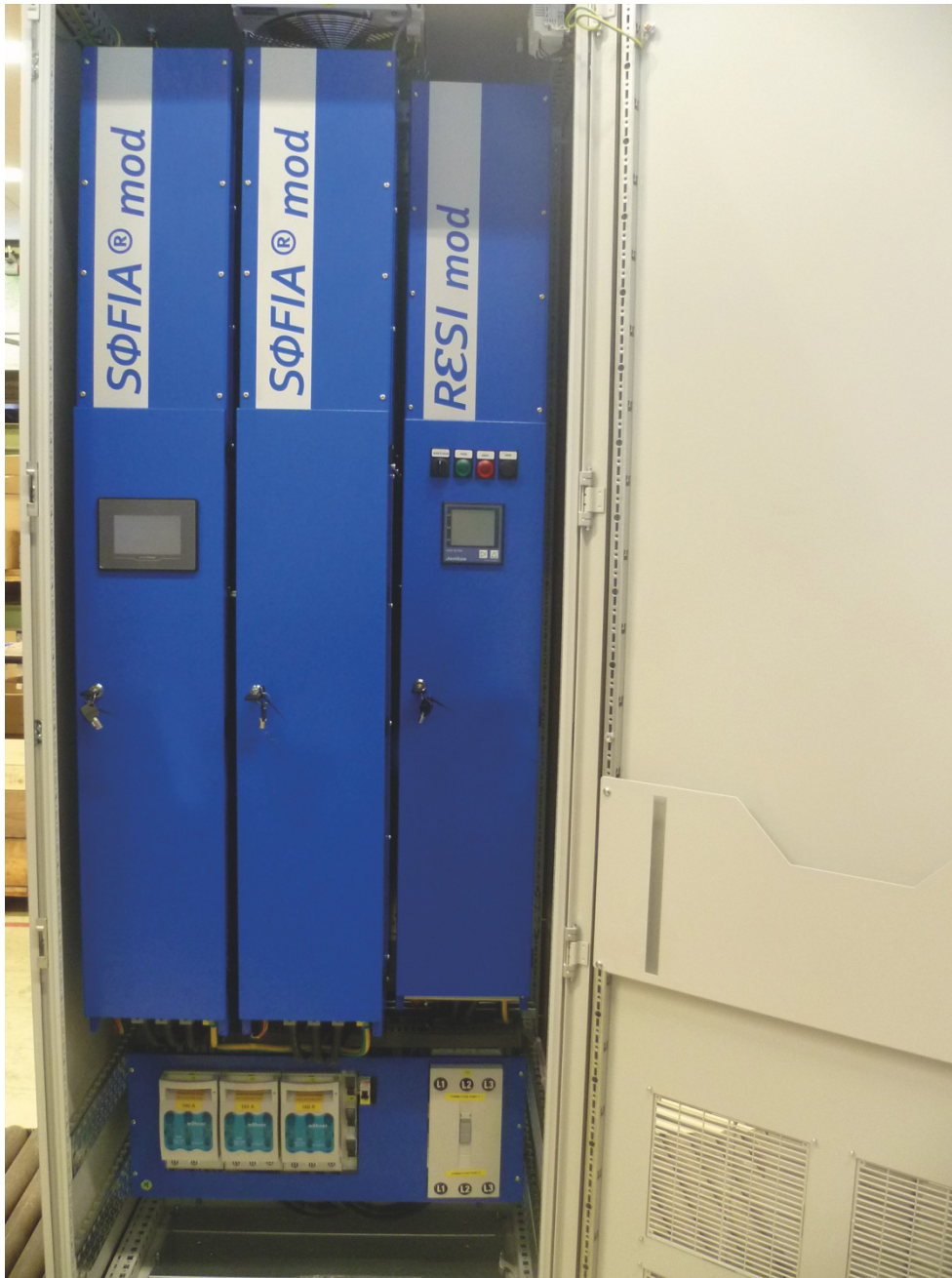
Figure 5: The GridClass®-Mod product line installed in a switch cabinet via plug and play. Centrally controlled broadband filtering of harmonics by SΦFIA®-Mod (filtering of the 5th, 7th, and 11th harmonics) in combination with the high-pass filter module RεSI-Mod.
